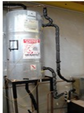
Indirect system – conventional Wetback plumbing
