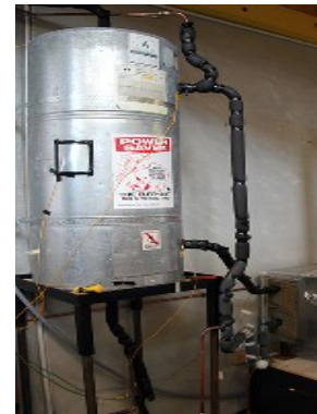
Indirect system – 'counterflow' Wetback plumbing.
